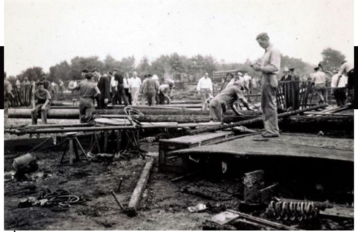
People examine debris and damage Photographed by James B. Hoye, 1988.134.3-O
